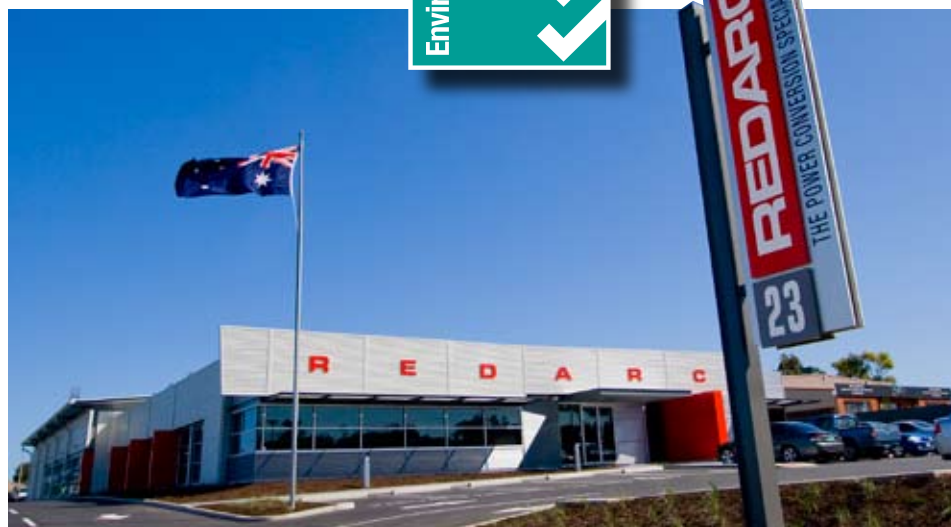
Redarc's new environmentally certified facility
