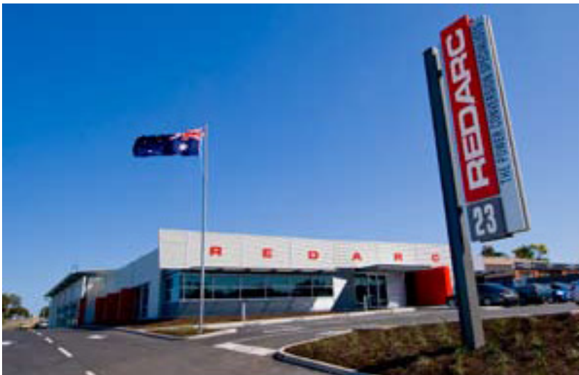
Redarc’s new environmentally certified facility
